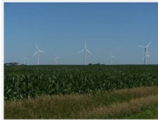
The wind farm, which began operation in December 2009, consists of 100 GE 1.5MW V150 turbines.
